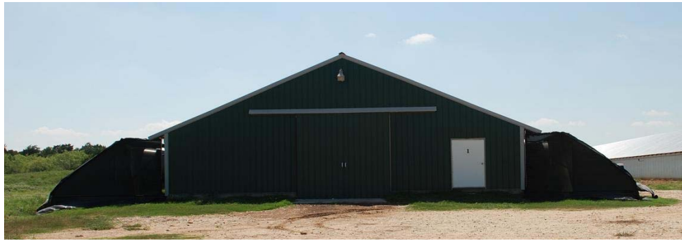
Figure 2. BioCurtain installations on poultry house
