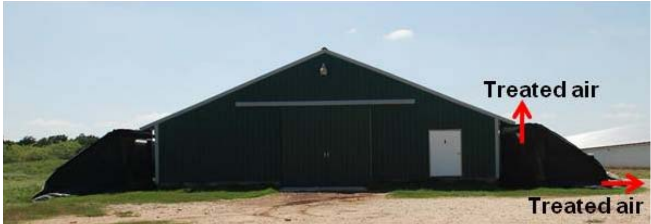
Figure 4. Biocurtain covering the entire exhaust area on both sides of the treatment house. Treated air leaves vertically and through the opening near the bottom corner of the structure. The BioCurtain™ functions by altering the aerodynamics of the air being exhausted from the barns by directing it toward the geotextile fabric and down into the bottom corner of the structure, where dust settles out of the air stream. The treated air is then exhausted out vertically and through the opening near the bottom corner of the structure (Figure 4). An EPI™ system was also installed inside the BioCurtain™ (Figure 5) enclosure to enhance the collection of suspended particles before the treated air leaves the structure.
