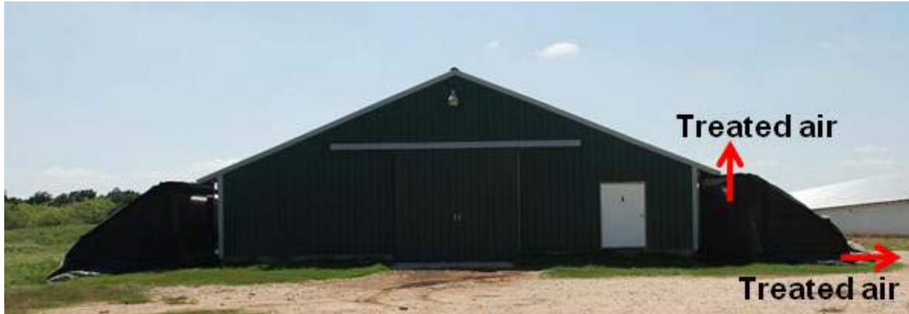
Figure 4. Biocurtain covering the entire exhaust area on both sides of the treatment house. Treated air leaves vertically and through the opening near the bottom corner of the structure. The BioCurtain™ functions by altering the aerodynamics of the air being exhausted from the barns by directing it toward the geotextile fabric and down into the bottom corner of the structure, where dust settles out of the air stream. The treated air is then exhausted out vertically and through the opening near the bottom corner of the structure (Figure 4). An EPI™ system was also installed inside the BioCurtain™ (Figure 5) enclosure to enhance the collection of suspended particles before the treated air leaves the structure.
